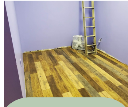
Flooring donation from LifeCycle Building Center
